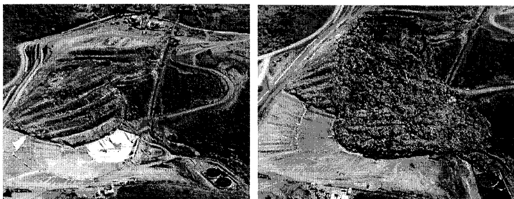
(a) Prior to failure
