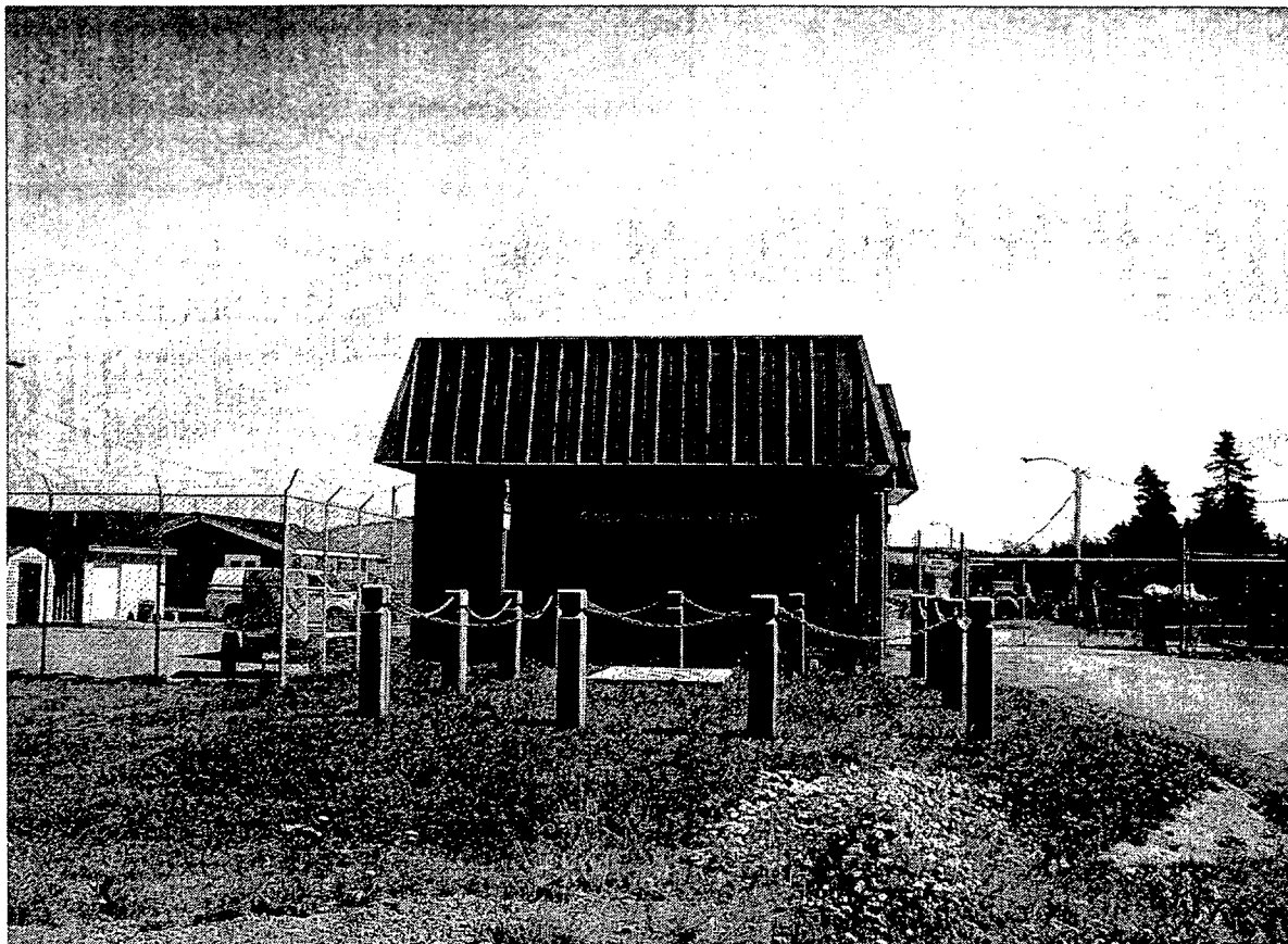
Figure 5.1. Goulds Pumping Station. This figure features the Goulds Pumping Station, once a source of severe flooding due to poorly designed storm sewers.
