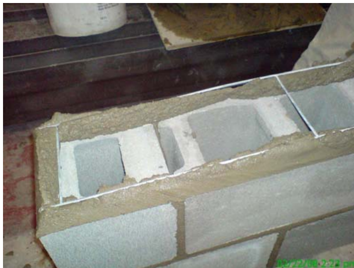
Figure 3.8: Steel Bed Joint Reinforcement in Wall-S
