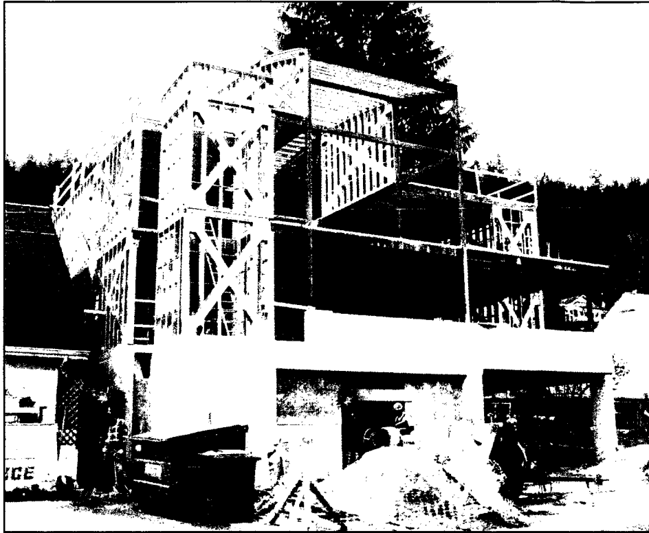
Figure 1.1: Example of building with weld connected strap braces ( Courtesy of CWMM Vancouver )
