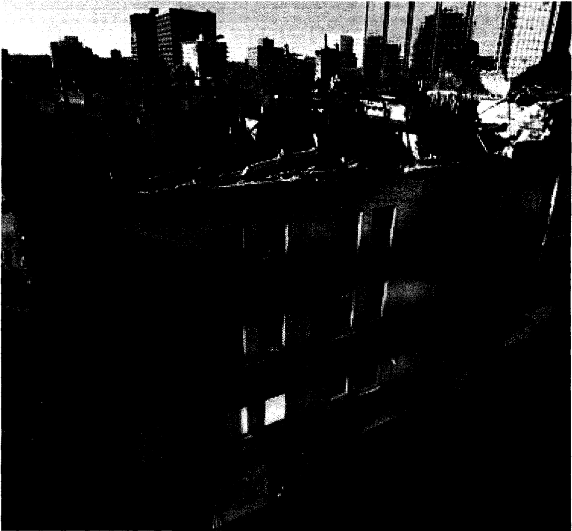
Arlington Apartment. Photo taken September 29, 2008. "Historic Downtown Apartment Finally gets its Demolition Order."
