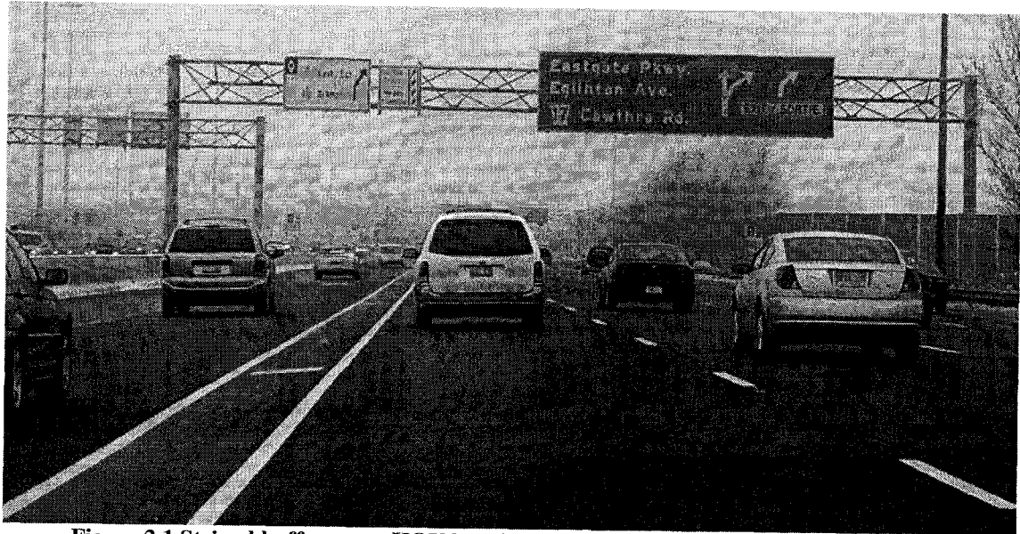
Figure 2.1 Striped buffer on an HOV lane in Mississauga, Ontario (Image Courtesy of: www.onthighways.com ).
