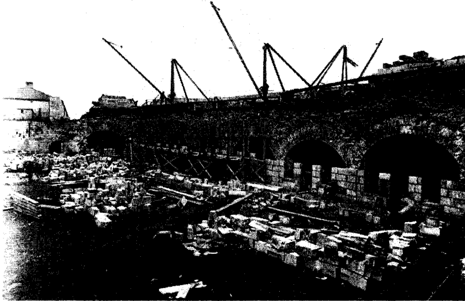
The Redoubt Casemates nearing completion during Way's reconstruction.
