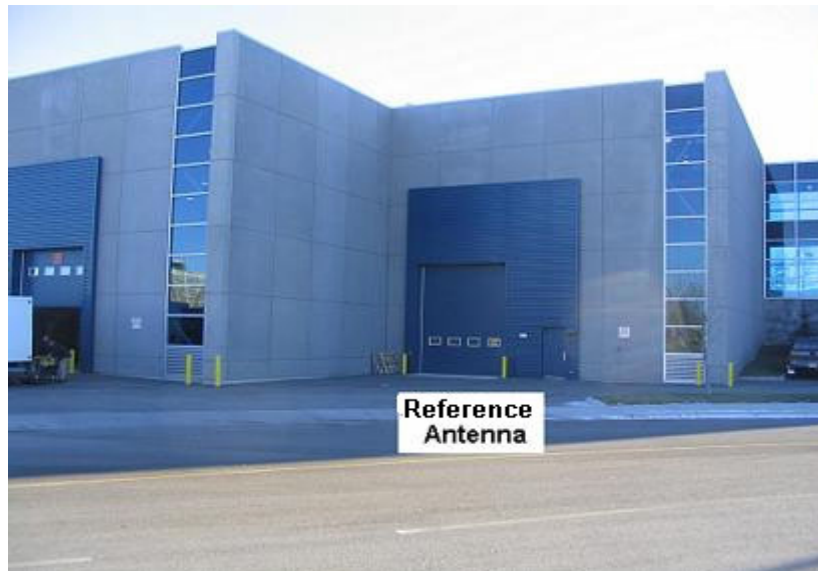
Figure 4.11: Surrounding Area for the Concrete Basement Test
