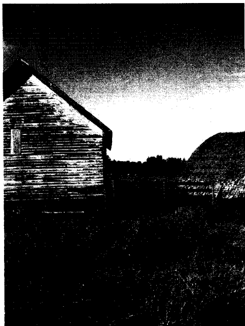
Remaining buildings moved from original Keephills townsite sit in a yard a few miles away
