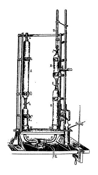
Figure 4. The blood gases apparatus of Ivan M. Sechenov. From I. Setchenow, "Beitrage zur Pneumatologie des Blutes" (1859) p. 295. For description see p. 77 opposite
