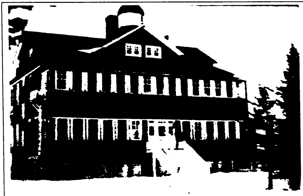
Plate 26: Sleeping Porches Added on To Sarcee Hospital (GA # NA 4397-25)
