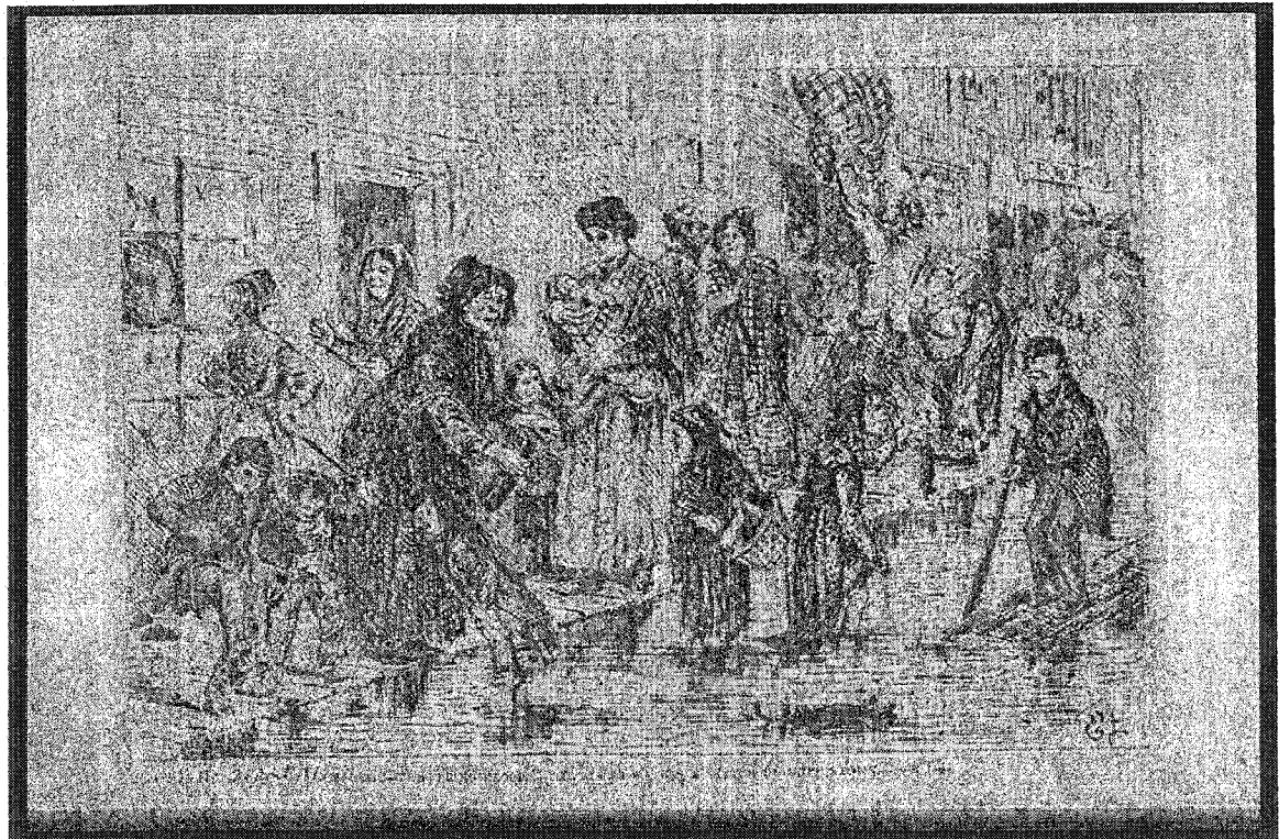
Figure 1.2 Seasonal flooding in Griffintown (Source: BNQ Albums Massicotte).
