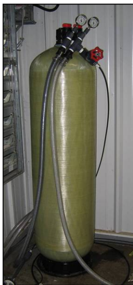
Figure 4-8 - Manganese dioxide filter used in Experiment III
