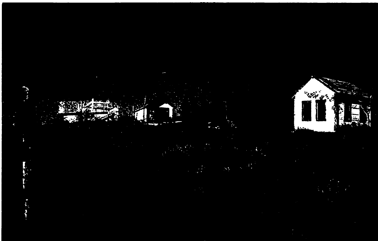
Fig. 2.27: Ruined gravehouses in cemetery at Canyon Creek, Yukon Territory.
