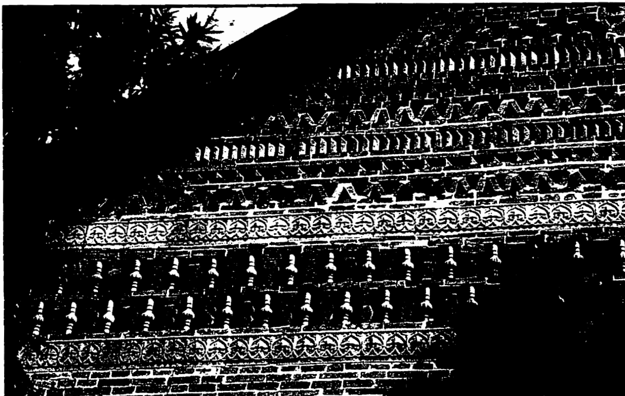
Fig. 5.17: Chamber of the Palace of the appanage princes, Uglich. Detail of brickwork incorporating floral, triangular and zig-zag motifs.
